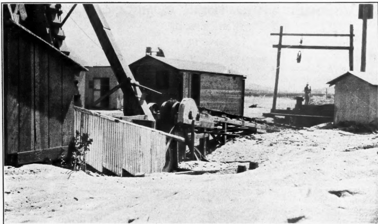
Conveyor, Crusher and Elevator at Plant No. 1
